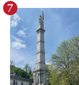
Civil War Monument 1916 • North Division Street & Highland Avenue
